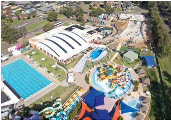
Myrtha Pools installation at Aquatopia in Western Sydney (and below).
